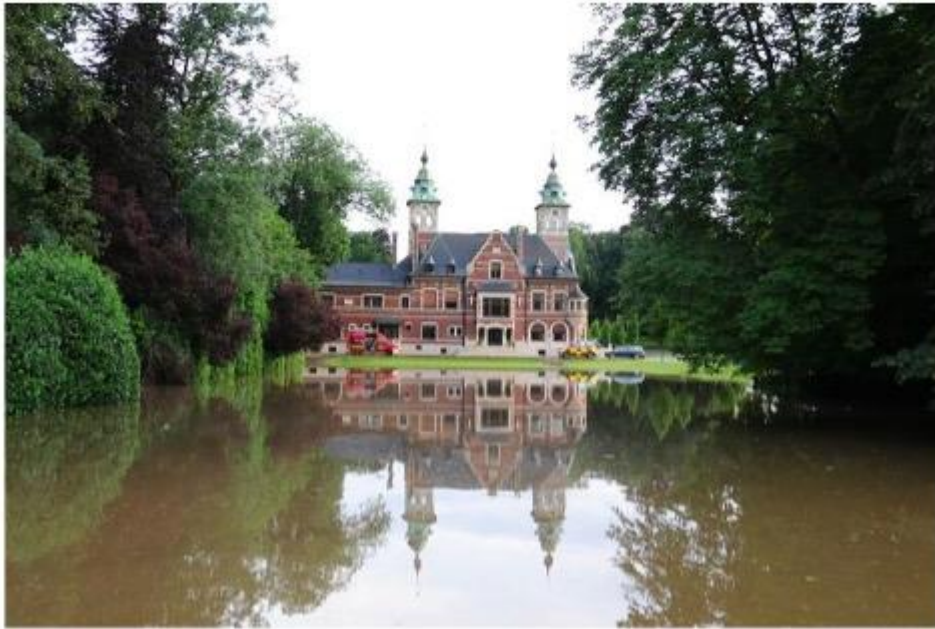
Castle Schotte threatens to flood. Heavy pumps have to be used to remove the water. Credit: Koen Baten
